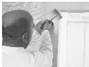
Figure 11: Protection of rough opening with StoGuard™ self-stick mesh and Sto Gold Fill® joint treatment. After placing the self-stick mesh into the rough opening and onto the face of the sheathing, apply Sto Gold Fill® over the mesh by spray or trowel, then trowel smooth.
