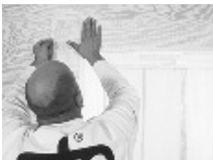
Figure 11: Protection of rough opening with StoGuard™ self-stick mesh and Sto Gold Fill® joint treatment. After placing the self-stick mesh into the rough opening and onto the face of the sheathing, apply Sto Gold Fill® over the mesh by spray or trowel, then trowel smooth.
