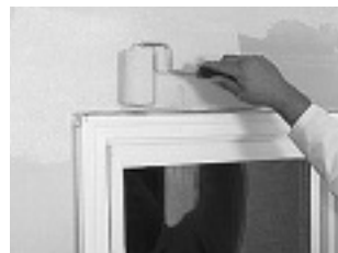
Figure 12: Application of waterproof coating. After treating rough openings, joints in sheathing, and inside and outside corners with Sto Gold Fill® joint treatment, apply Sto Gold Coat® or Sto EmeraldCoat™, as appropriate, to the entire wall surface. Apply by spray or roller.
