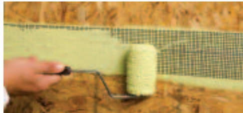
StoGuard Fabric on OSB
